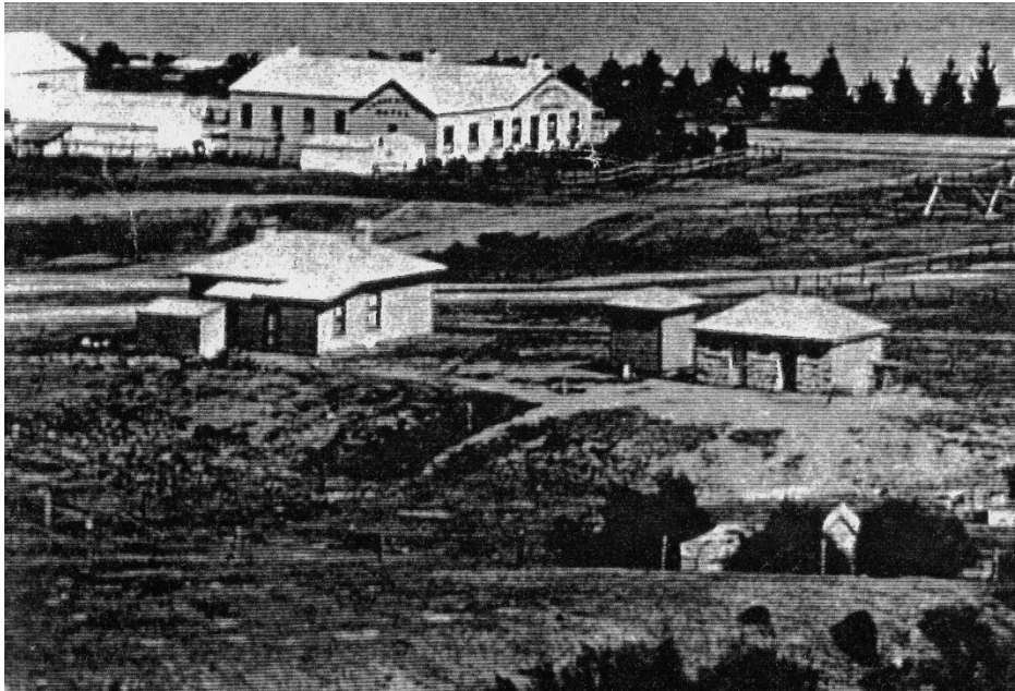
This photo is from around 1890 and shows the first Residence and Station, the single-cell block and the stables. In the background is the Commercial Hotel built by William Allan in 1885.
